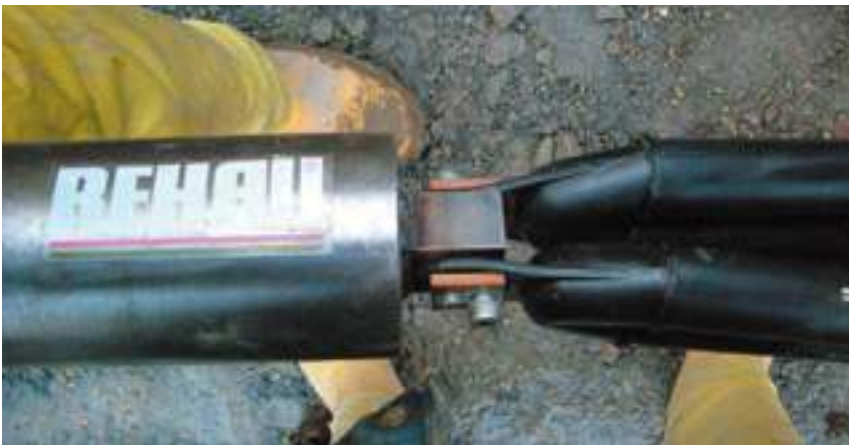
Fig. 51: Fastening the probe weight
