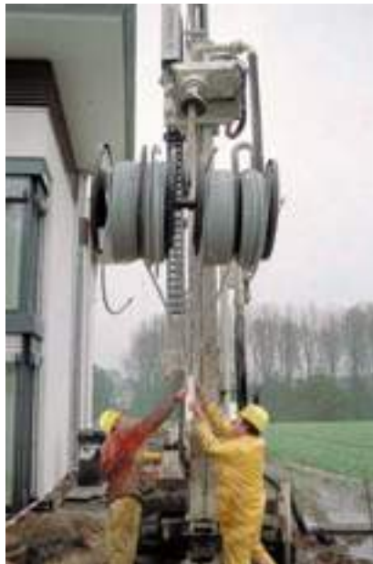
Fig. 4: Installation of a RAUGEO probe Xa
