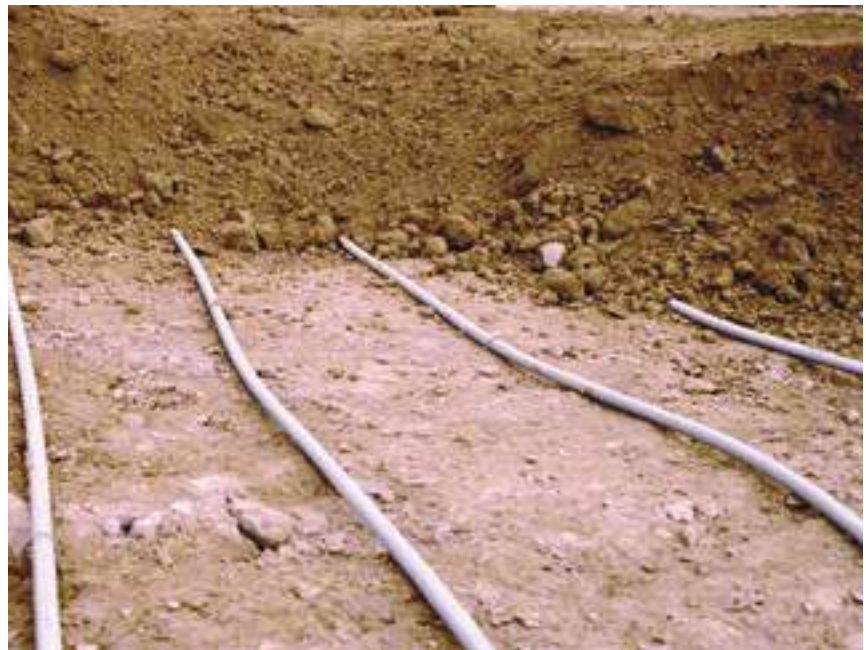
Fig. 10: RAUGEO collect Xa building site photo
