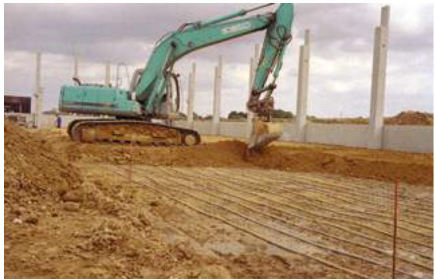
Fig. 43: Open cast laying
