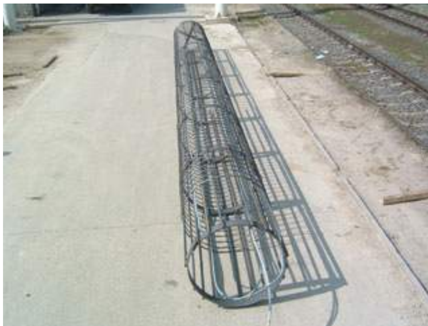
Fig. 14: REHAU energy pile
