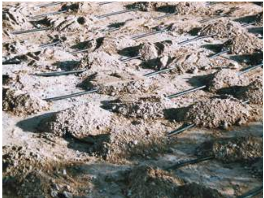
Fig. 12: RAUGEO collect PE100 building site photo
