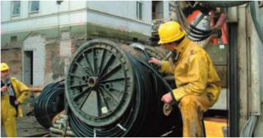
Fig. 50: Filling the probe pipes with water
