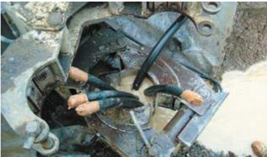
Fig. 52: Compacting the annular gap with an aggregate
