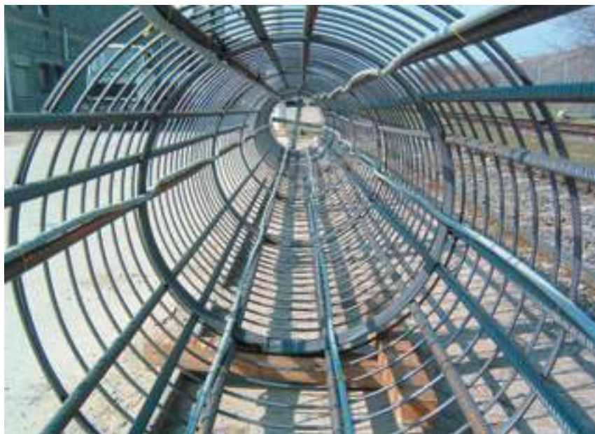
Fig. 54: Energy pile pipe laying
