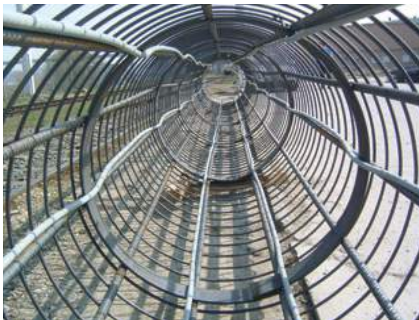
Fig. 15: Inside view of REHAU energy pile
